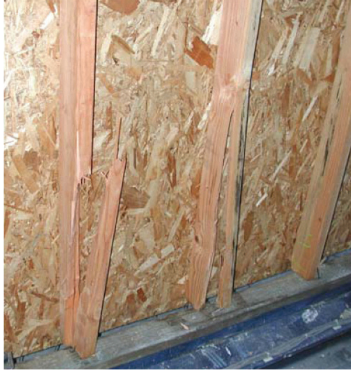
Figure 6 - Damage State 3 for Walls with OSB/Plywood Sheathing (System #50): Replacement of Entire Wall (from Gatto and Uang 2002).
