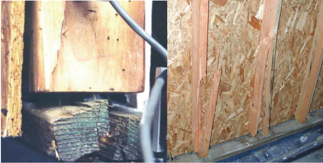
Figure 11 - Damage State 3 for Walls Incorporating Stucco as Exterior Finish: Replacement of Entire Wall (from Gatto and Uang 2002).
