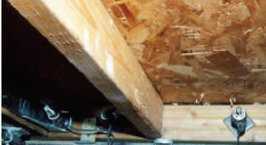
Figure 4 - Damage State 1 for Walls with OSB/Plywood Sheathing (System #50): Slight Separation of OSB/Plywood from Framing (from Pardoen et al. 2002).
